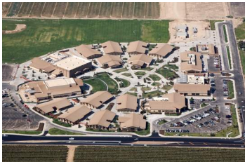
MIRA MONTE HIGH SCHOOL New Construction
