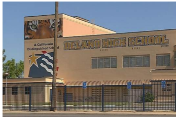
DELANO HIGH SCHOOL New Construction
