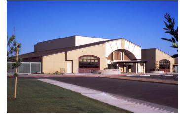
GOLDEN VALLEY HIGH SCHOOL New Construction
