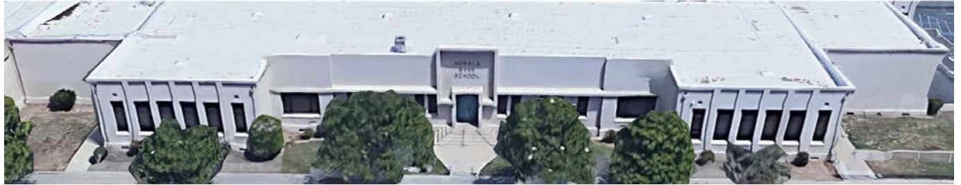
Exterior elevation photograph, looking North, taken: July 26, 2018 using Google Earth
