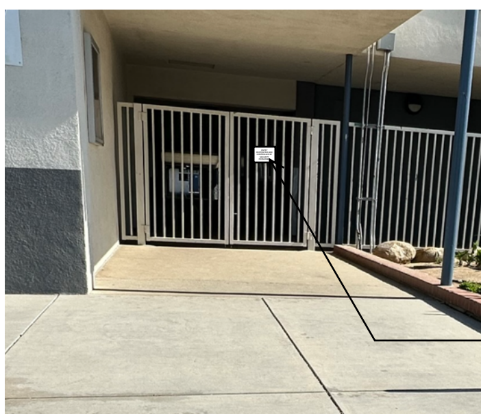
EXISTING FENCE WEST OF BUILDING "B" GATE ACCESSIBILITY COMPLIANCE PER 2022 CBC 11B-04.1, EXCEPTION 1.
