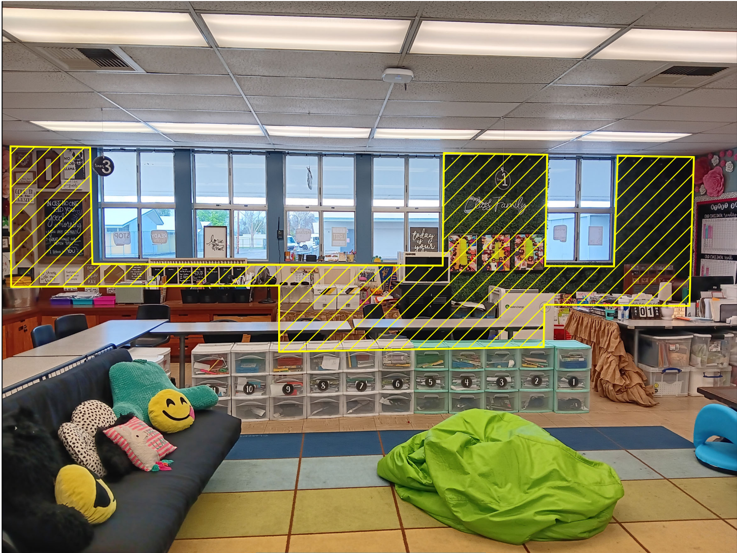
ROOM 29 NORTH WALL
