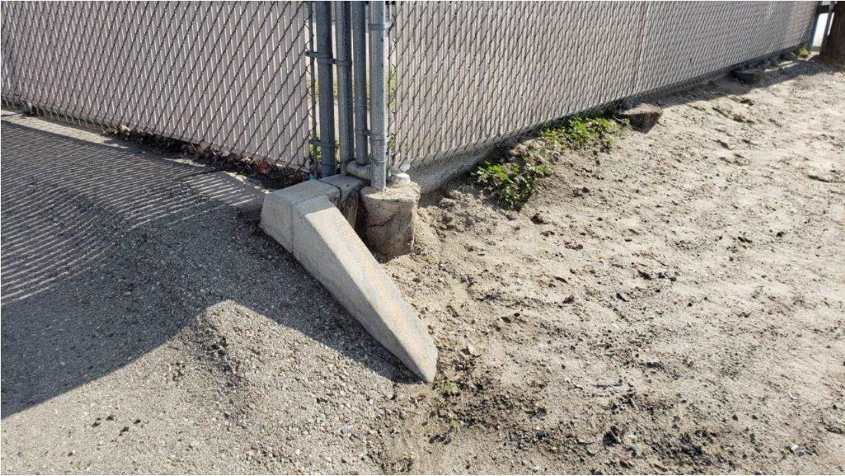
South exit – south side condition
