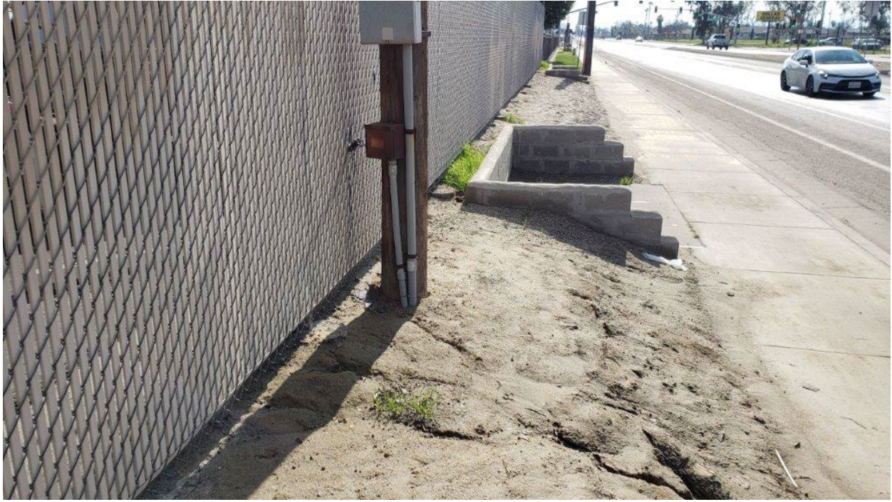
Utility pole with possible underground conduits to be aware of
