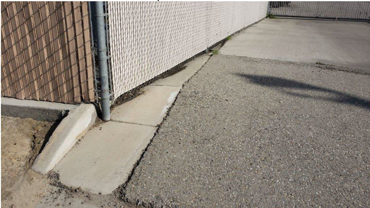
South exit – north side condition
