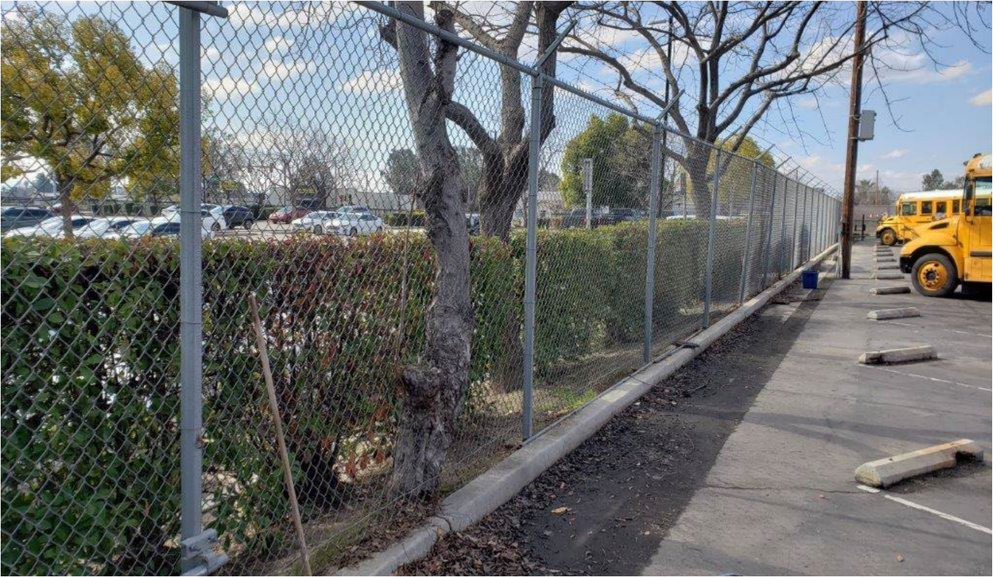
Tree within chain link fencing to be removed by contractors.
