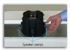
**STEP 9** - Drop the speaker wire down from the empty tile hole in the ceiling and connect it to the speaker. Remove the insulation from the end of the wires. While pushing the plastic tab to open the terminal insert the bare wire into the terminal hole and release the tab. Connect the red wire to the red terminal and the black wire to the black terminal.
