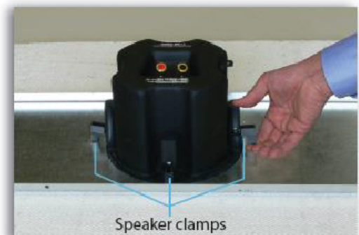
Rear view of a properly mounted speaker with tile bridge. Note three of the speaker clamps are visible.
